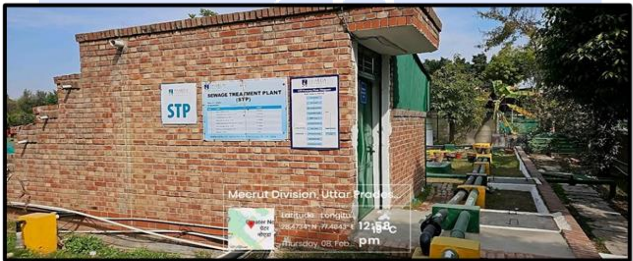
Fig. 38: Sewage Treatment Plant
