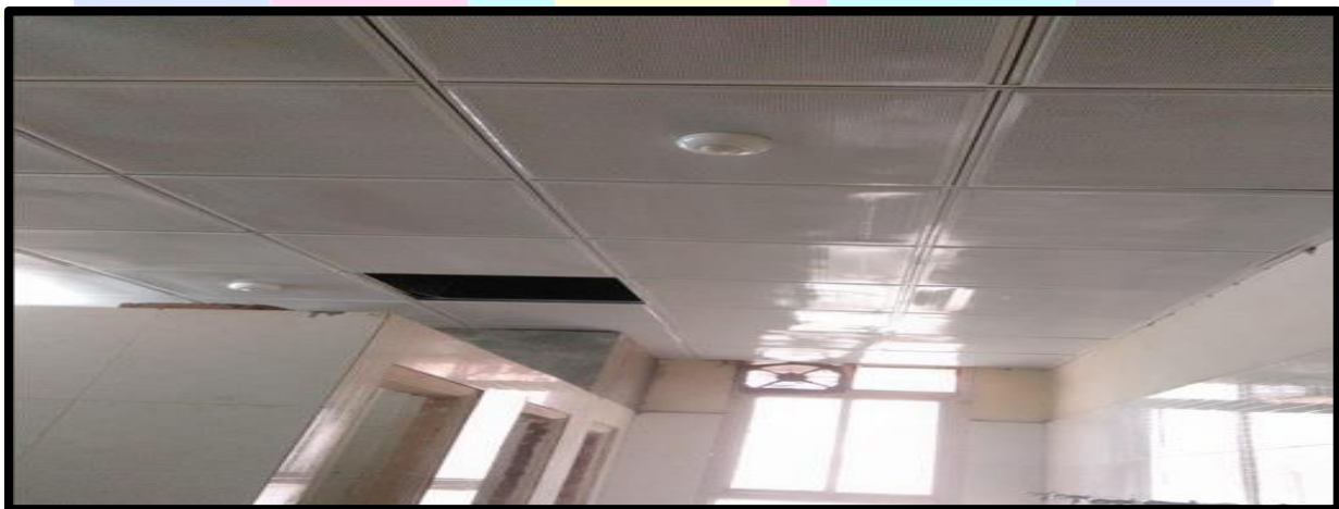
Fig. 7: Sensor Lights in Washroom
