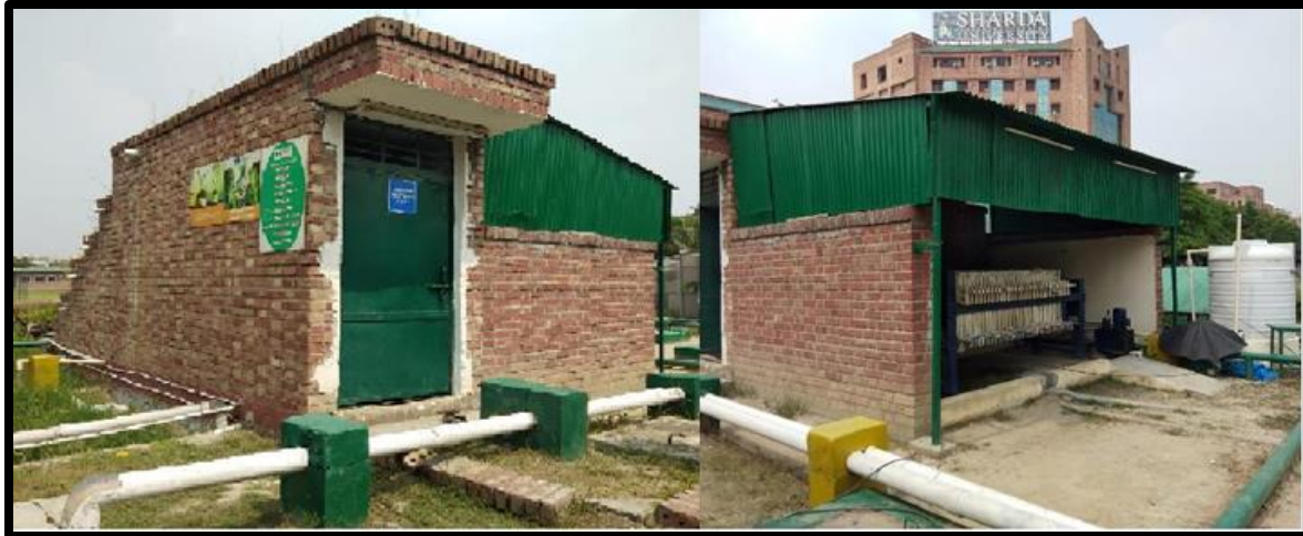
Fig. 12: Sewage Treatment Plant (STP)
